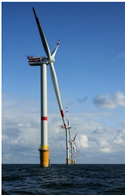
Figure 1: Newly constructed wind turbines.
