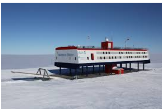
Neumayer III Station
