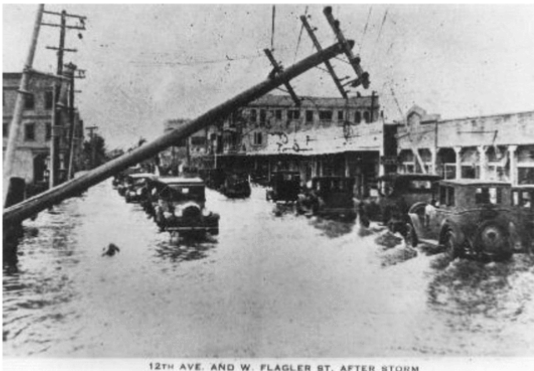
Damage in downtown Miami after the 1926 hurricane
